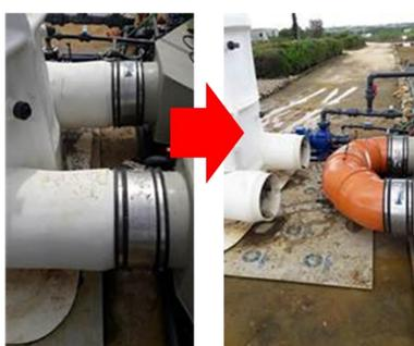
Figure 2 – U turn connection used to replace one VAL column
